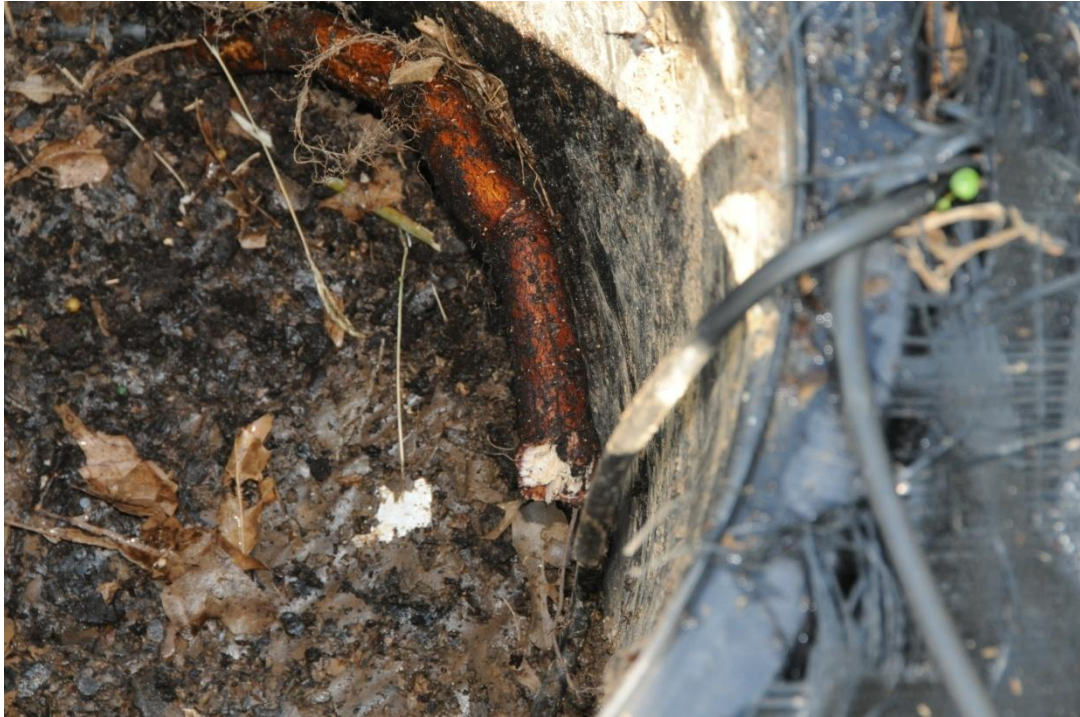
Figure 10. A large root which had to be cut before removal of the RootTrapper®-in-Pot Insert from the socket pot.
