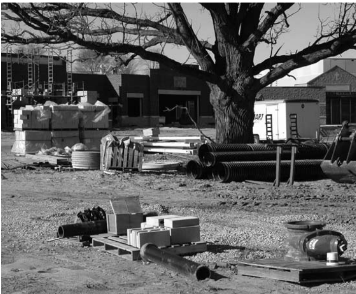
Figure 3a. An assortment of materials was stored near the base of the tree and substantial compaction of the soil occurred.
