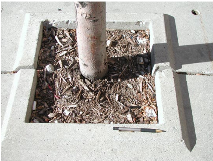
Figure 1. These trees were planted into openings about four by five feet. But once planted, concrete units were positioned over most of the surface leaving an exposed soil area of only about 16 by 20 inches. Scale is provided by the ball pen on the concrete.
