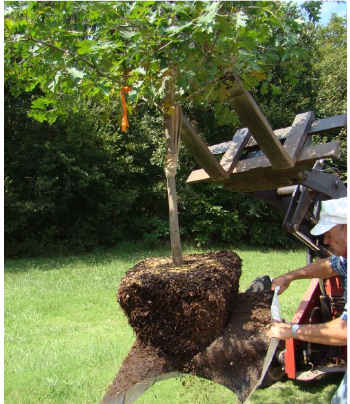
Figure 4. Once on the job site, the white RootTrapper® fabric is easily removed and can be returned to the nursery and used again.
